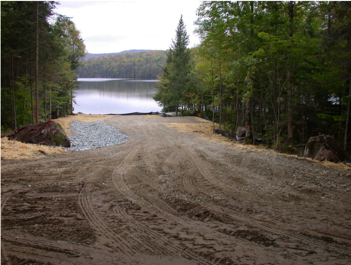
Millsfield Pond Public Boat Access Facility, Millsfield, NH
